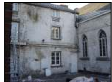
Before shot of the interior courtyard.
